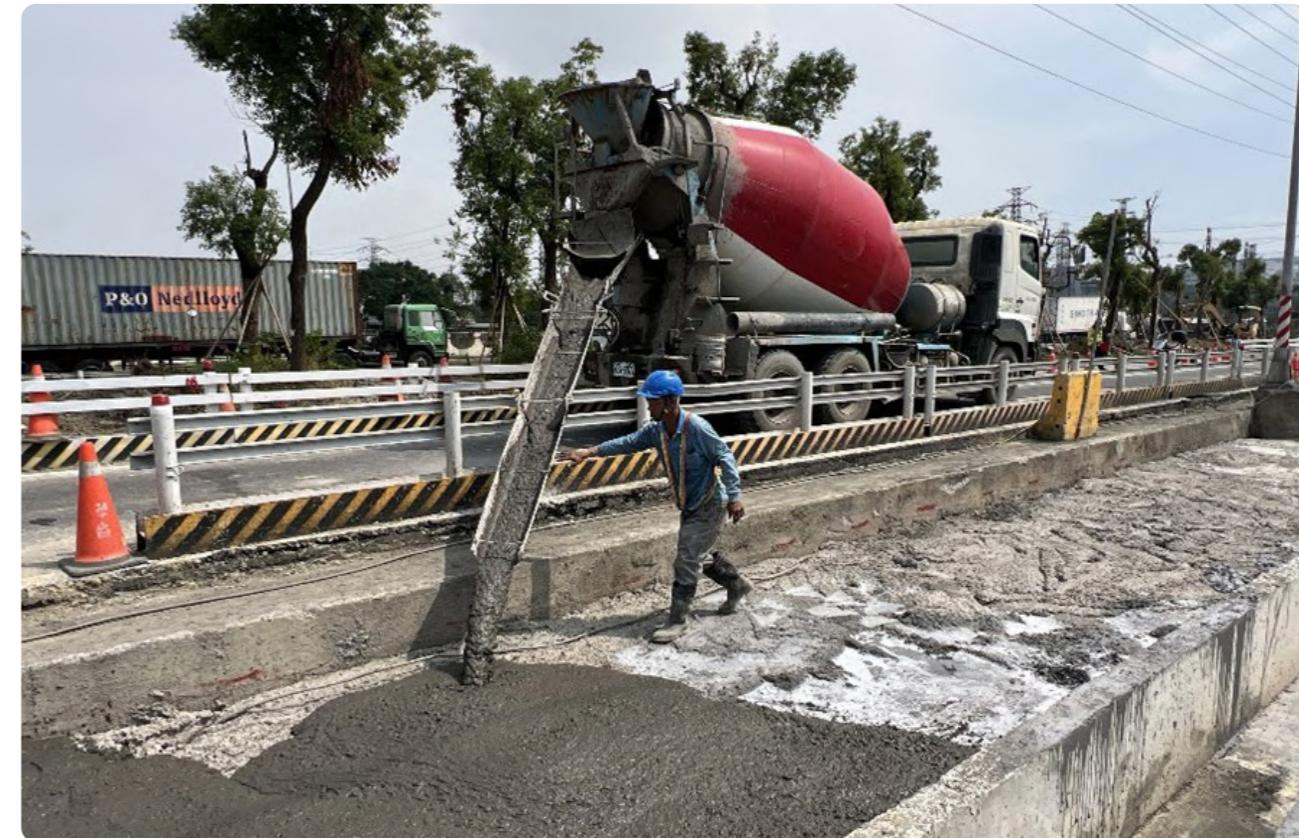
Pouring of Controlled Low Strength Material (CLSM) from Recycled Aggregate
