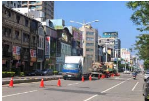
Love River sewage interception system pipeline inspection and improvement
