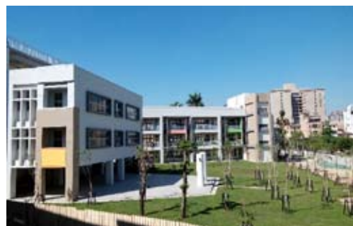
Phase 2 of School Building Reconstruction at Dingjin Junior High School in Sanmin District
