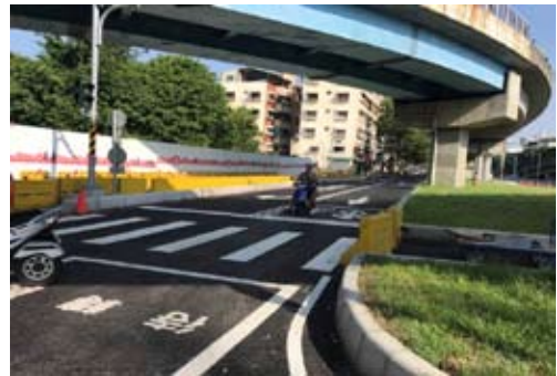
Zuoying underground sewer filling-in and restoration project
