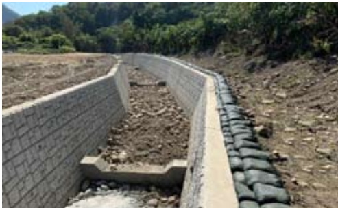
Liouguei District Laonong Village Jhangfen Creek third-phase improvement project
