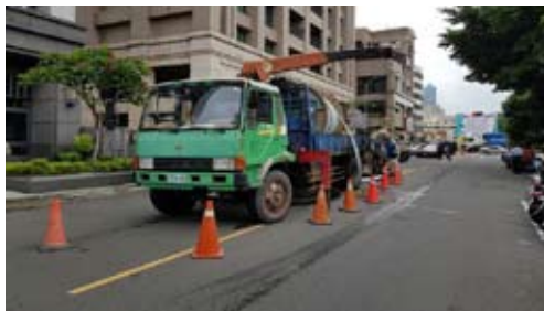
Kaohsiung City's sewer system maintenance open-ended project
