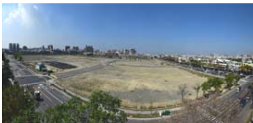
Completed work of Phase-89 Urban Land Consolidation Zone
