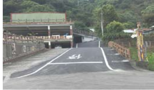
Tribal Road Improvement
