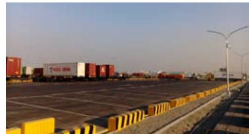
A public car park for heavy vehicles at special warehouse zone A completed in phase I
