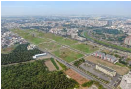
Completed work of Phase-87 Urban Land Consolidation Zone
