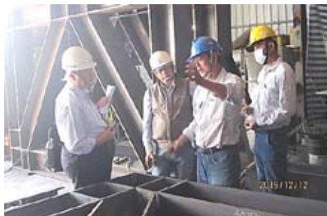
Inspecting steel structure material quality at the steel plant
