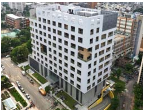
Construction of Integrated Long-term Care Center for the Elderly
