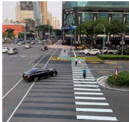
Pedestrian refuge islands at Minzhu-Jhongjheng road junction
