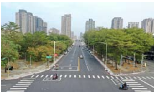
Demolition (or leveling) of three-dimensional facilities under Kaohsiung Railway Underground Project – Qinghai bridge and four culvert facilities at Hebian Street
