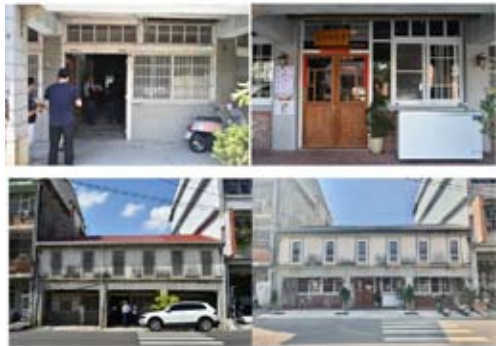
Successful revitalization case – No.197 Yong'an Road, Meinong District (Meinong Tankaotang)
