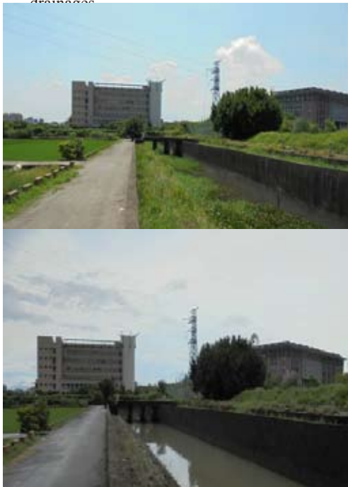
Channel dredging work
