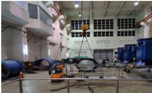
Love River Surrounding Water Environment Plan – Sewer Sluice Gate Replacement
