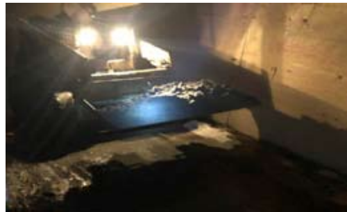
Rainwater sewer dredging work
