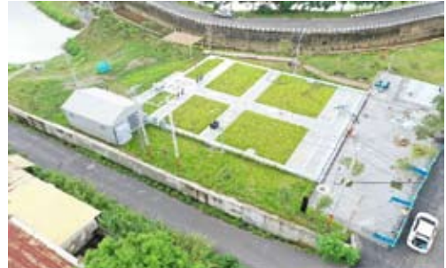
Fongshan Canal water quality improvement and purification plant test operation completed
