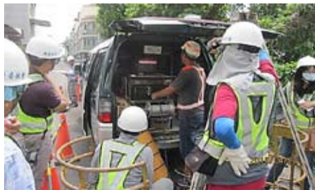
Taking core samples at the work site
