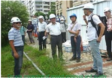
On-site inspection of project progress and quality
