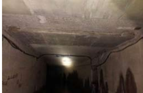
Rainwater sewer repair work
