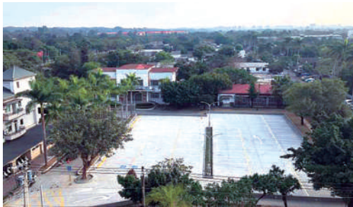
Huangpu Village Public Parking Lot
