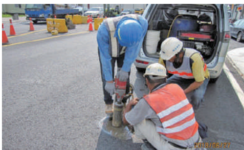
Taking core samples at the work site
