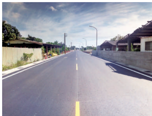
Lujhu District Kaohsiung County Road No. 11 Widening Project
