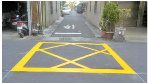
Installation of criss-cross lines
