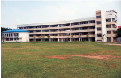
Daliao District Chaoliao Junior High School Construction Project
