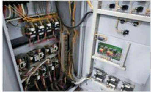
Control Panel Renewal
