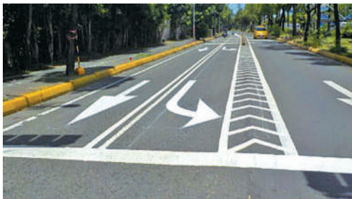
Installation of direction lines and channelizing lines
