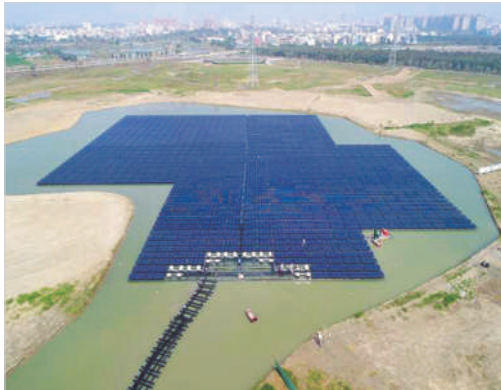
Dianbao River Area B flood detention pond floating photovoltaic system
