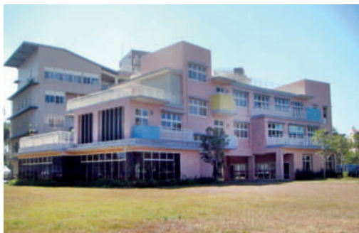
Yancheng District Yancheng Junior High School Construction Project
