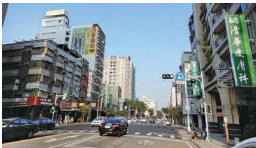
Underground conduit lines at the intersection of Sanduo Road and Syueyuan Road in Lingya District
