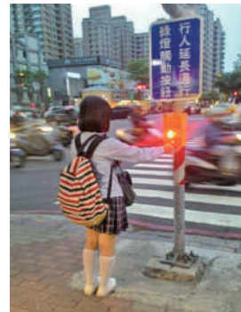
Delay-time actuated traffic signal controls
