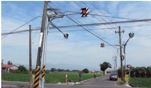
Solar-powered warning lights
