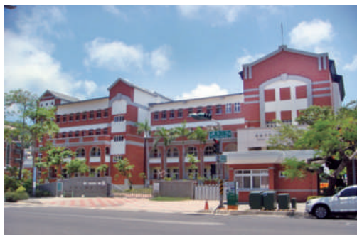
Gushan District Gushan Elementary School Demolition and Construction Project
