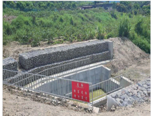
Dashan Bridge drainage embankment repair project in Cising Village, Tianliao District
