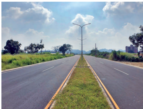
National Highway No. 10 Yanchao Interchange Extension for Kaohsiung County Road No. 46 to Connect Route 186A Project (first tender)
