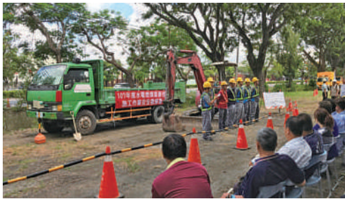
Utility lines excavation construction safety observation activity
