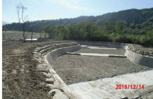
Wucitan Longhu Mountain Kaohsiung City DF021 potential mudslide river renovate project
