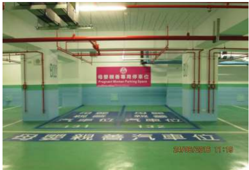
The underground parking lot of Foxconn's Software R&D Building at Kaohsiung Software Technology Park in Cianjhen District
