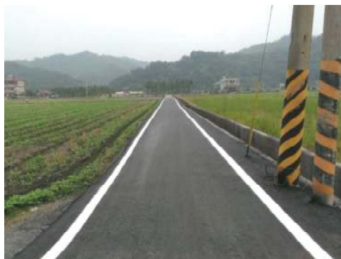
Important agricultural road and irrigation canal improvement construction project in the agricultural land consolidation area
