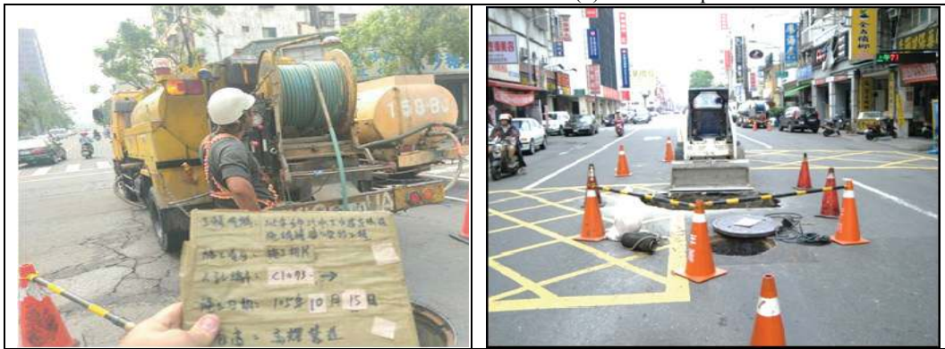
Inspection and improvement of the city's sewage system
