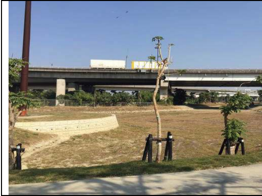
Lowering of the greenbelt and creating a small flood detention area near the Kaohsiung City freeway interchange ramp (Dingjin Interchange)
