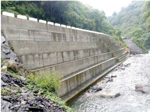
Maolin District Musheng River revetment repair project
