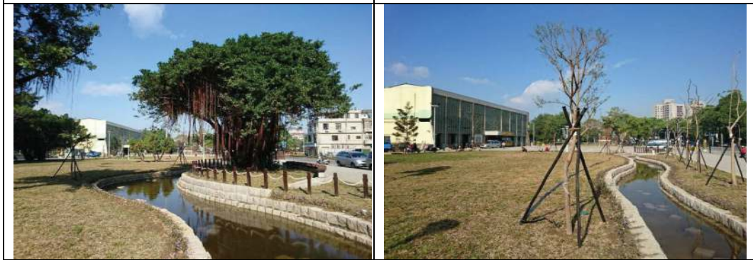
Caogong Canal Phase 6 (Anning St. to Fuxing St.) Project
