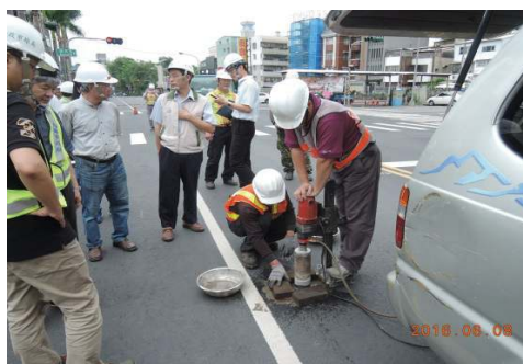
Taking core samples at the work site
