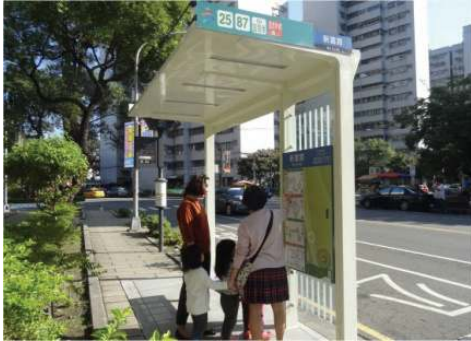
A cantilever style bus waiting shelter
