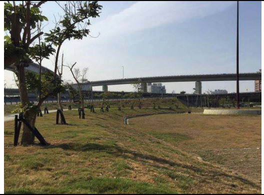
Lowering of the greenbelt and creating a small flood detention area near the Kaohsiung City freeway interchange ramp (Dingjin Interchange)
