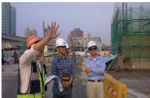
On-site inspection of project progress and quality
