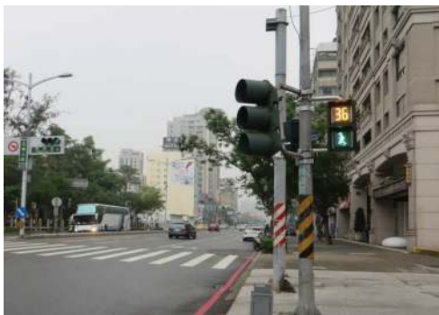
The newly installed pedestrian signal at the intersection of Wufu Road and Yingsyong Road in Cianjin District
