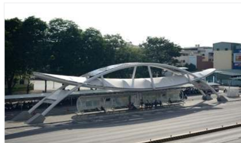
Siaogang Transfer Station
