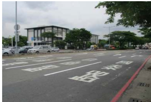
The markings of road names and directional indications on Zhongjheng 1st Road (Jianjyun Road - Chengcing Road) in Lingya District
