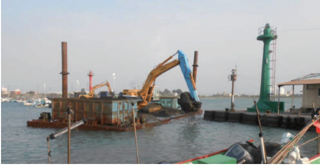
Dredging project in Yongsin Harbor
