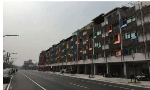
Restore gas explosion area outcome (kaisyuan Rd.1)
