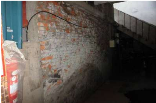
Before house repair
