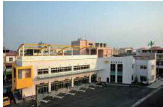
Cishan Transfer Station
