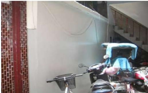
After house repair
