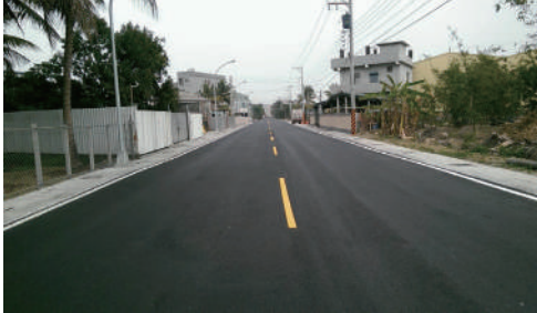
Widening project of Jiashu Road (Kaohsiung Country Road No. 36-2) in Ciaotou (Lilin E. Road – Kaohsiung Country Road No. 30)
