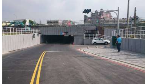
Culvert widening project for Hougang Lane
