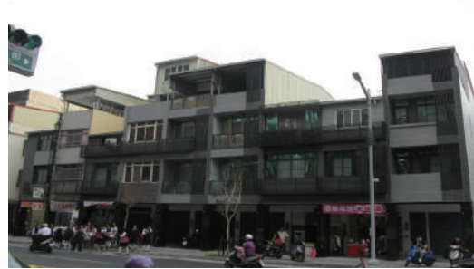
Restore gas explosion area outcome (Sanduo Rd. )
