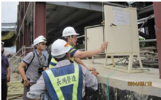
On-site verification of construction progress and quality
