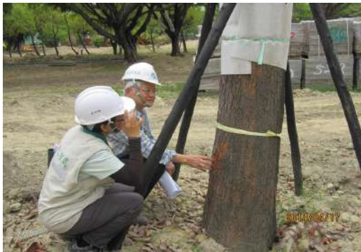
On-site verification of construction progress and quality
