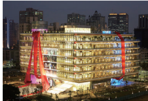
The new main Public Library
