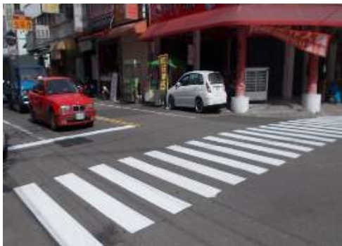
Pedestrian-crossing marking additionally painted on Jhongsia Road in Yanchao District
