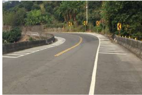
New Channelizing-Speed hump on Sanhe Road in Dashi District
