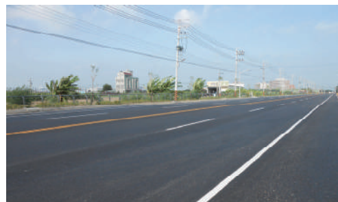
Widening project of Kaohsiung Country Road No. 68 in Daliao
