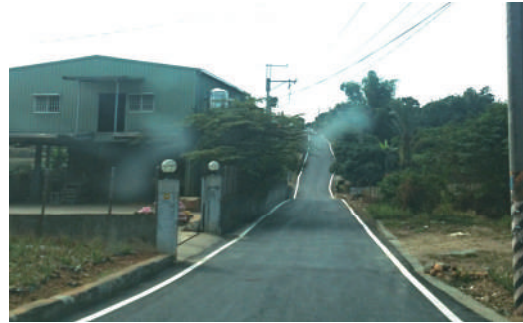
Maintenance of rural roads in Shui-An Village, Dashu District
