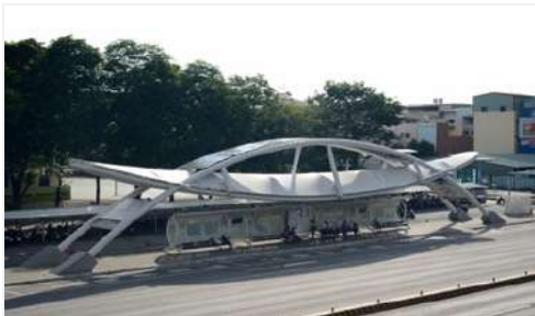
Siaogang Transfer Station
