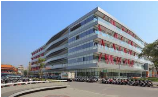
Fongshan Administration Center Construction Project)
