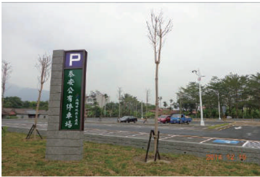
Tai-an public parking lot
