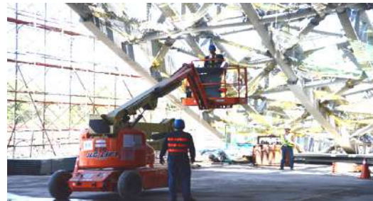
Observation of construction and steel structure fall prevention
