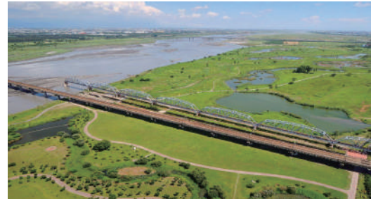
Dashu Old Railroad Bridge Kaohsiung – en
