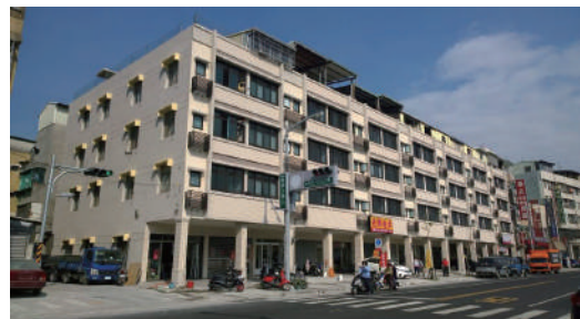
Restore gas explosion area outcome (kaisyuan Rd.3)
