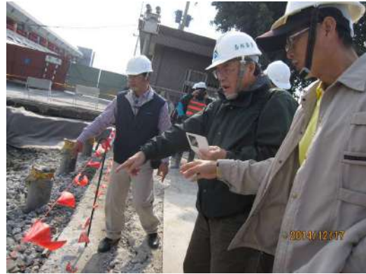
On-site verification of construction progress and quality
