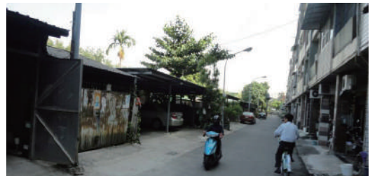
Pre-construction of Siaogang Daling Steel Spur railway
