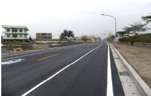
Widening project of Kaohsiung Country Road No. 79 in Daliao
