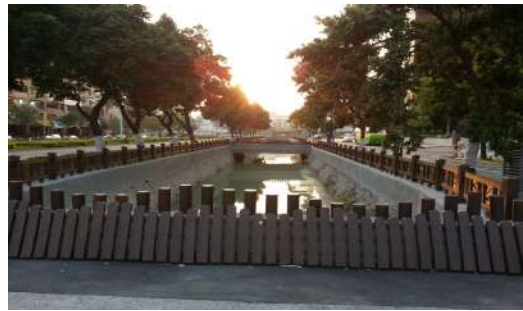
Restoration of Minsheng, Sihwei, and Jianjyun Village Great Drains
