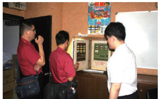
Inspecting fire-safety equipment.
