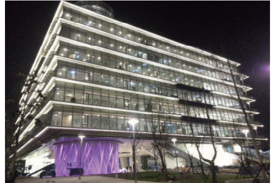
Kaohsiung Public Library Headquarters Construction Project
