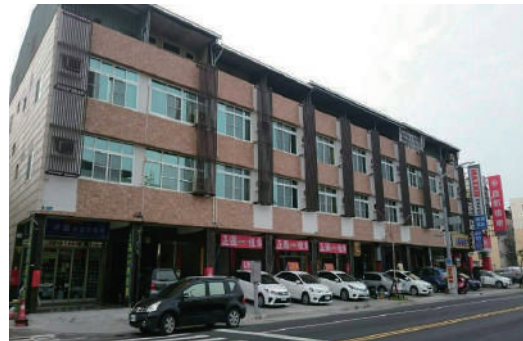
Restore gas explosion area outcome (kaisyuan Rd.2)
