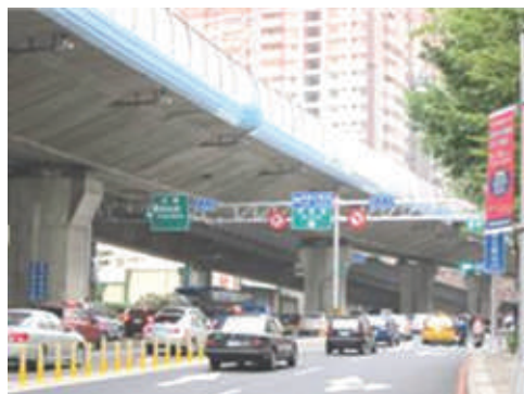
Improvement of Zihyou Road exit ramp – 2
