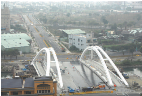
A 30-meter parkway was constructed in 42 nd and 68 th redevelopment zones.
