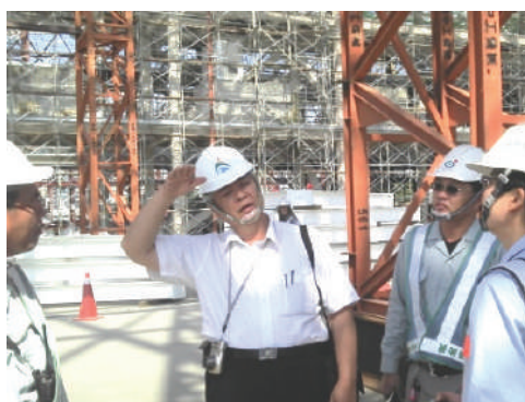
On-site inspection of construction progress and quality
