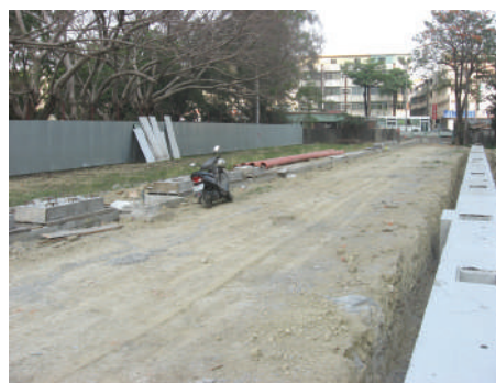
Construction and site surfacing work of the 73 rd Urban Redevelopment Zone
