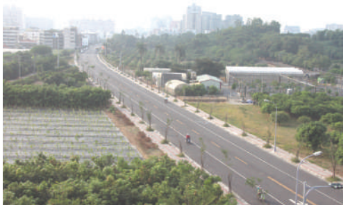
Construction of Fongcing Urban Land Consolidation is completed
