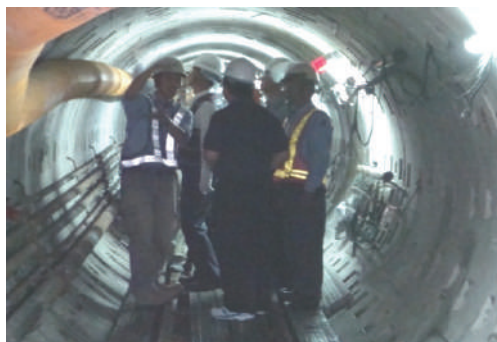
On-site inspection of construction progress and quality
