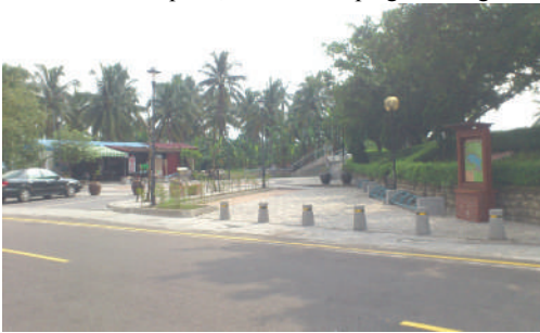
Improvement of lakeside surroundings of Jhongjheng Lake in Meinong
