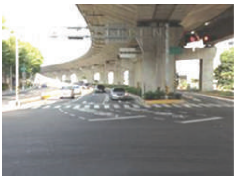
Improvement of Zihyou Road exit ramp – 1
