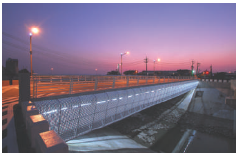
Photo showing the completion of the reconstruction project of the new Guanyin Bridge at Agongdian River in Gangshan District (Gangyan Bridge)
