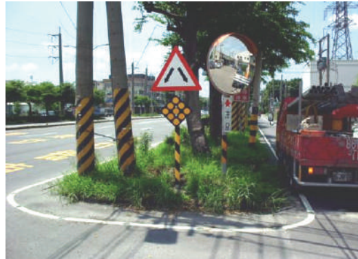
Convex mirror erected between Fongren Road/ Rensin Street in Renwu District
