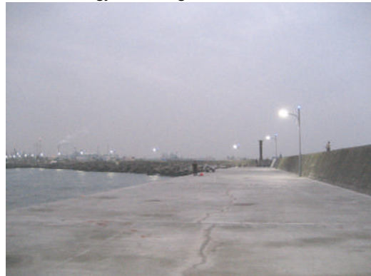
Streetlamp installation construction for Zhongyun Fishing Port
