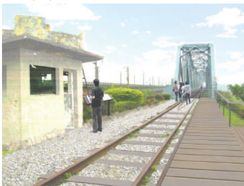
Revitalization of national monument – Dash Old Railroad Bridge
