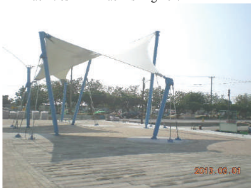
Improvement construction for facilities on wharf of Eziliao Fishing Port
