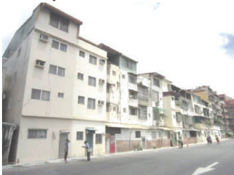
Old buildings located at Lane 238, Guangyuan Road, Fongshan District – Before transformation
