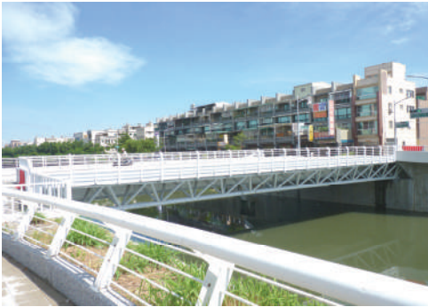
Photo showing the completion of the reconstruction project of Ming Feng Bridge in Cianjhen District
