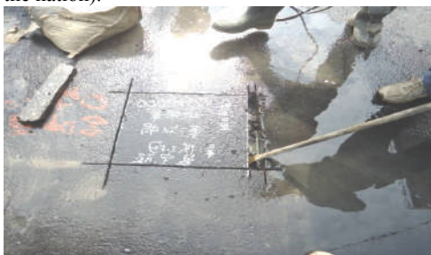
On-site inspection of construction progress and quality
