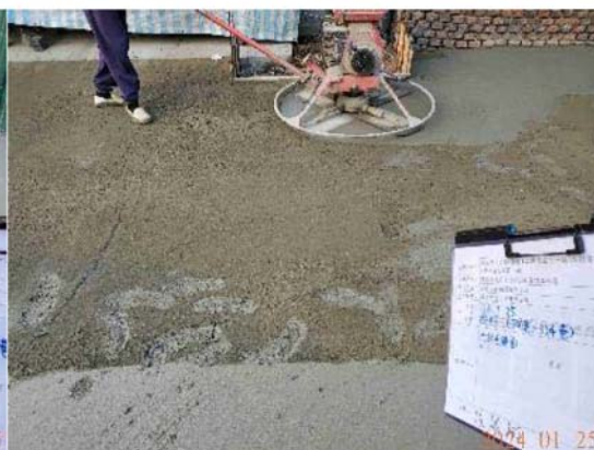
(6)面層澆置後粉光拉毛
