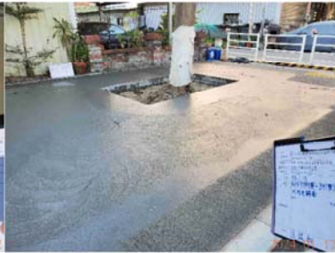
(6)面層澆置後粉光拉毛
