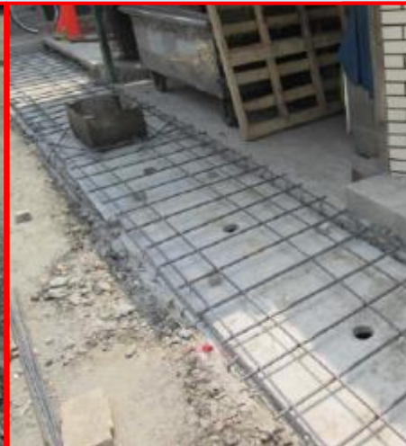
頂板鋼筋綁紮
