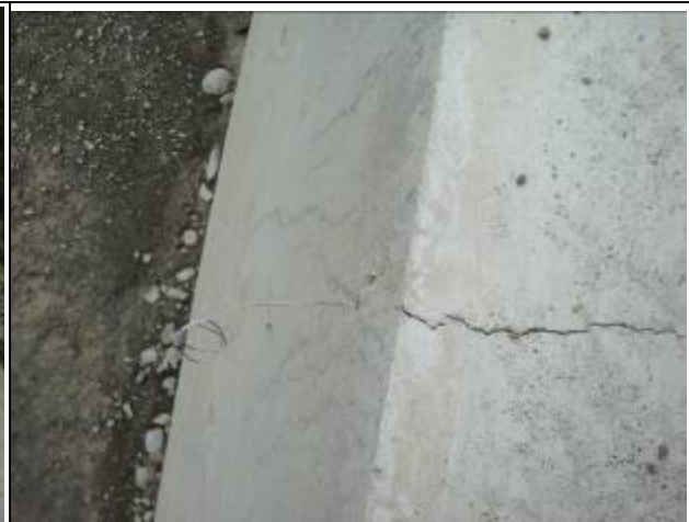
擋土牆頂橫向表面裂縫
