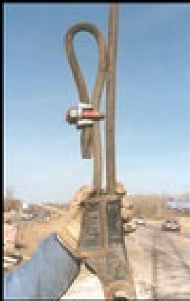
Single Grip, Single Saddle Wire Rope Clamp (One Single Saddle with U-bolt)
